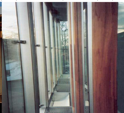
FIG.10 Interior View of Arag Tower shaft facade, Dusseldorf (Oesterle et al, 2001)
