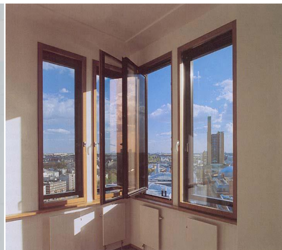
Fig.5 a box window at Berlin Postdamer Platz building (Oesterle et al, 2001)
